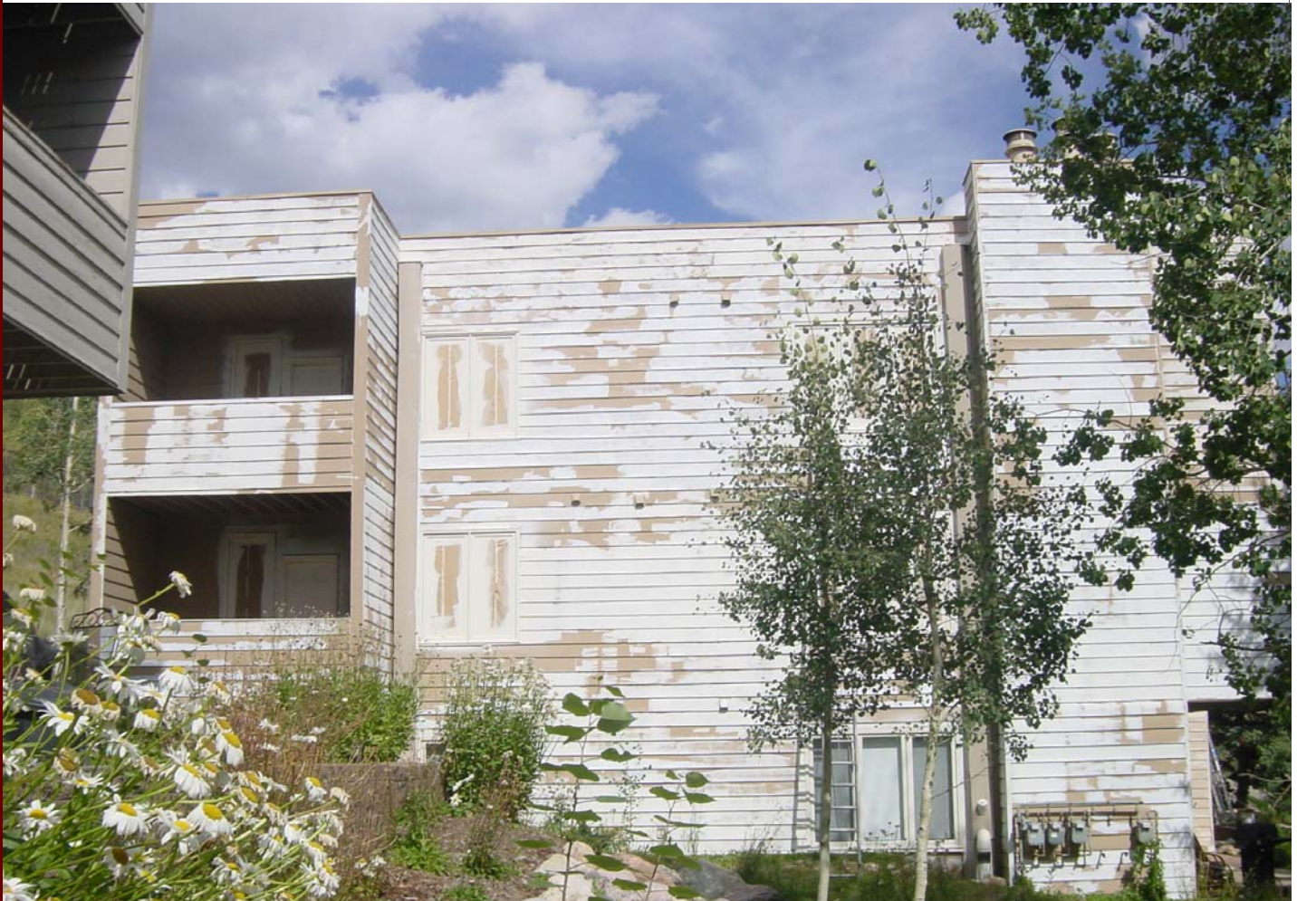
Fall 2007 Exterior Painting Included Priming of Woodwork
